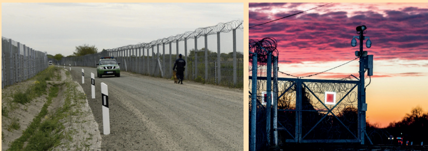
Figure 25. Two-layer security barrier, patrol roads and surveillance systems at the border between Hungary and Serbia Source: Hungarian border police
